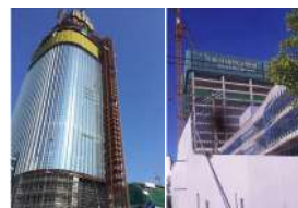
PosMAC Steel Curtain Wall (Construction case of rectangular forming bar)
